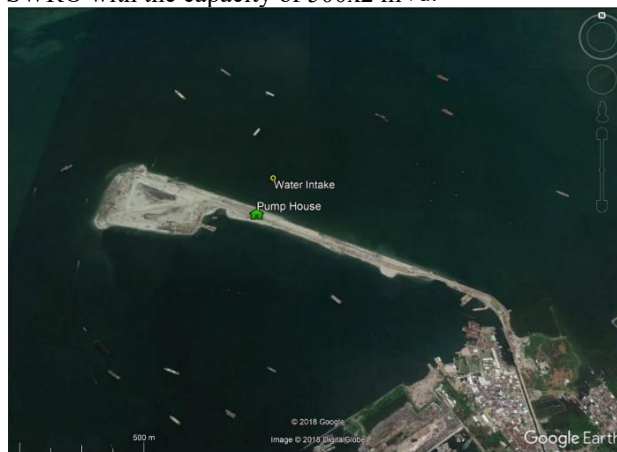
Fig. 9. The location of the water intake point (yellow dot). The distance between the water intake point to the pump house is approximately 250 meters.
