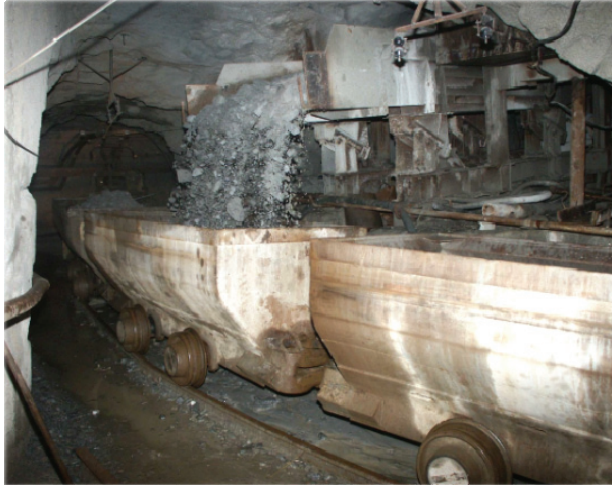
Fig. 2. Vibratory feeder of the VPR-4m type for the ore drawing and feeding from the panel to the wagons.
