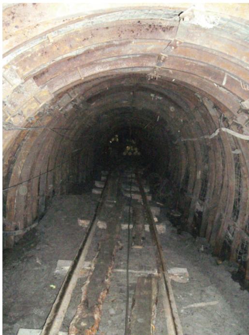
Fig. 4. Boundary entry condition in the most unfavorable area for its maintenance (the area of rock inrush).
