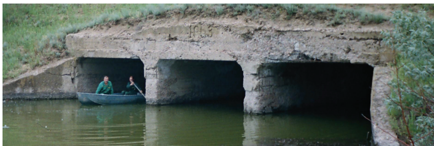
Fig. 9. Appearance of culvert.
