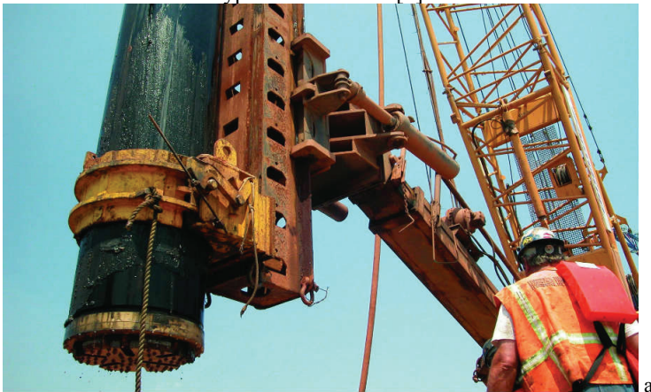
Fig. 12. Start of drilling for a pile of 1016 mm system Symmetrix.
