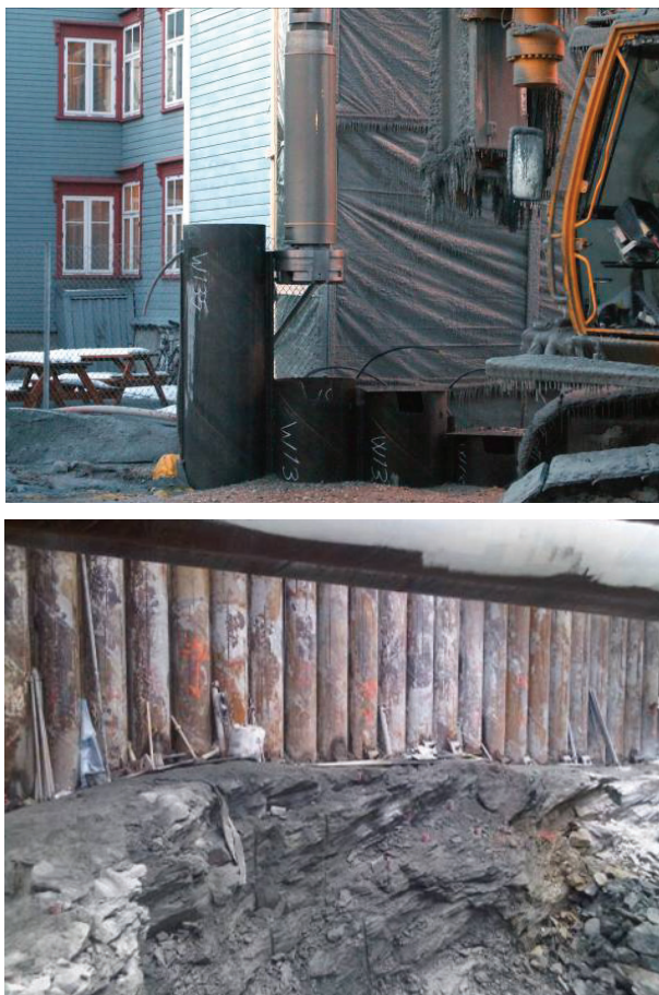
Fig. 16. Tunnel construction in Trondheim using pile wall technology.
