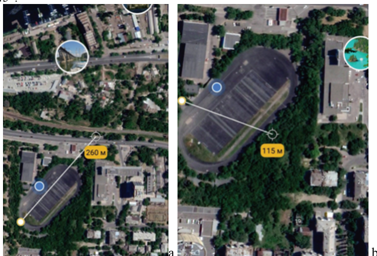
Fig. 6 a, b. Gully bottom construction along the 6th Strilkovoi Divizii str. with sports facilities of the “Slavtych” sports complex.
