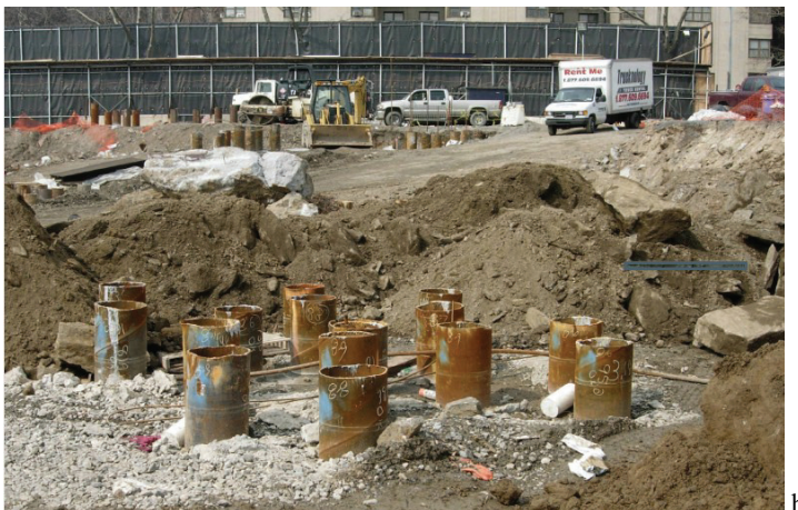
Fig. 12. End of drilling for a pile of 1016 mm system Symmetrix.
