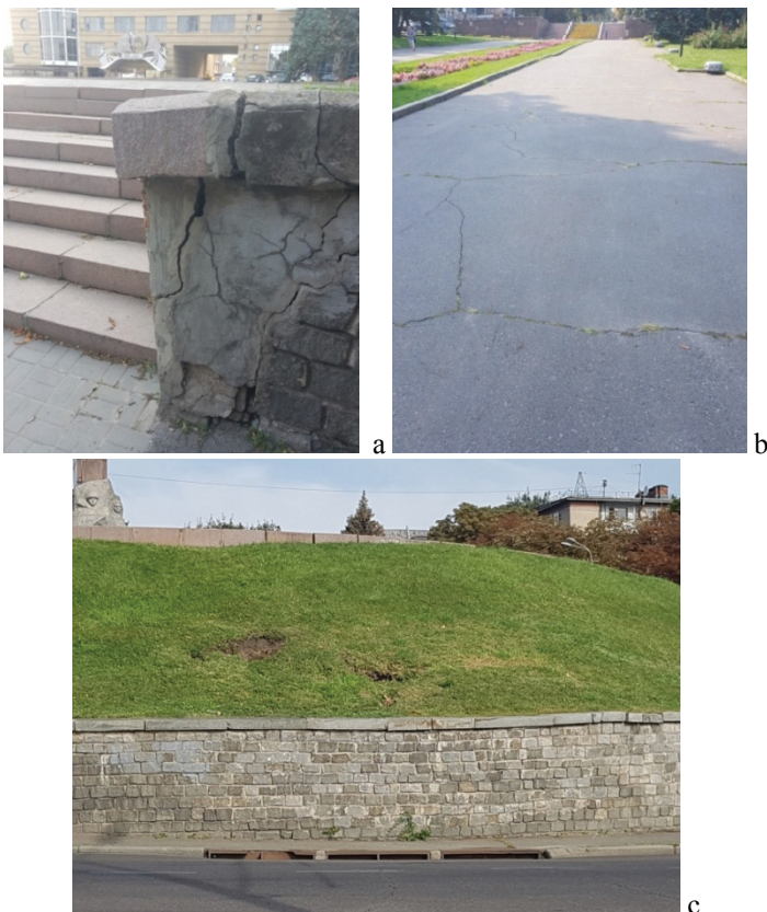
Fig. 2 a, b, c. Traces of parapet deformations in the area of the Glory Monument.
