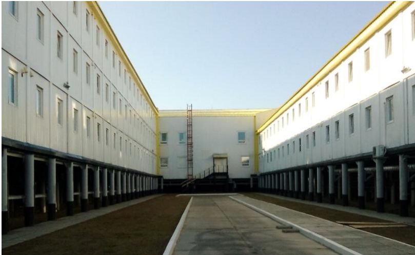
Fig. 4. Structures erected on steel shell pile
