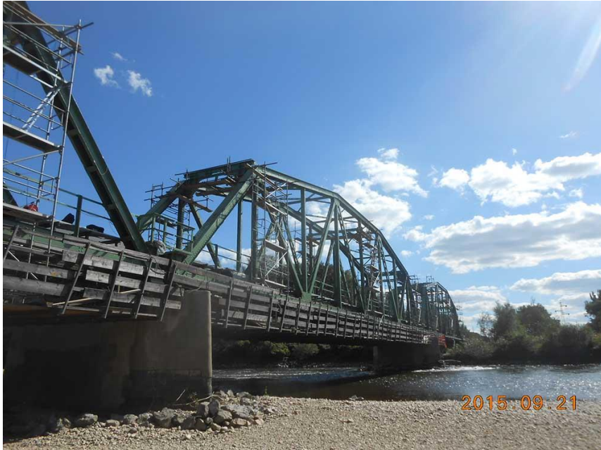
Fig 1. Railway bridge during reconstruction (Source: IMK Institute for metal structures).
