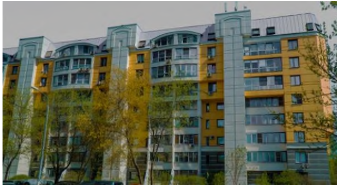
Fig. 3. First industrial generation residential building of the period 1956-1968 after reconstruction.
