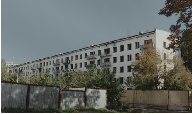
Fig. 2. First industrial generation residential building of the period 1956-1968 before reconstruction.
