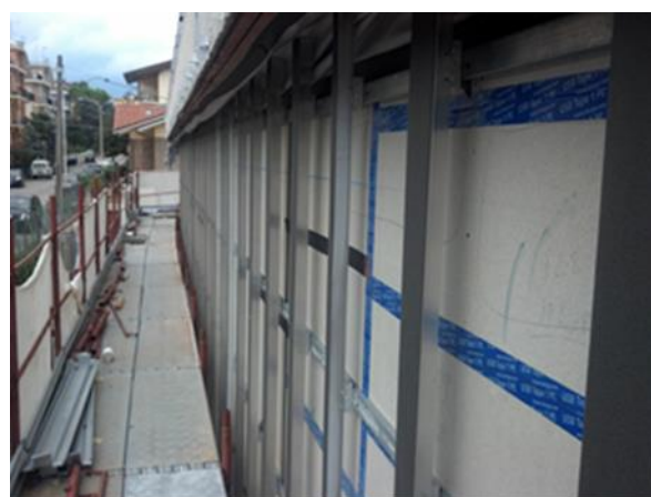
Fig. 8. Ventilated wall structure.
