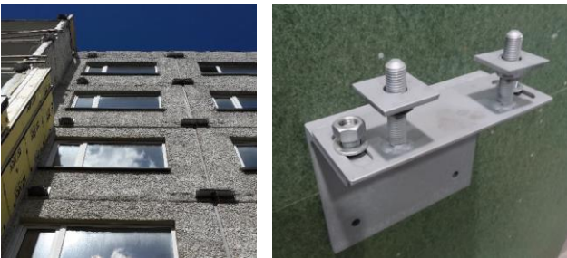
Fig. 9. Adjustable fixings (hangers) of wall module panels.
