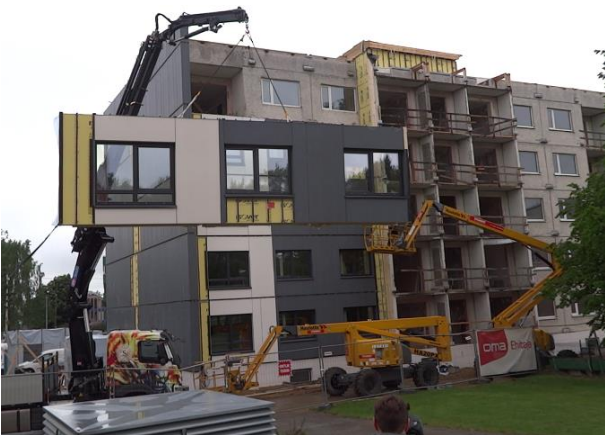
Fig. 8. Installation of the prefabricated wall element.
