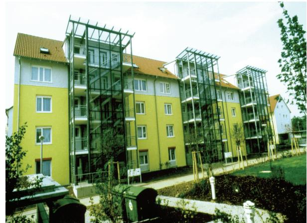
**Fig. 4.** Photos of the multi-family house in Stuttgart-Stammheim realised with external staircases.
