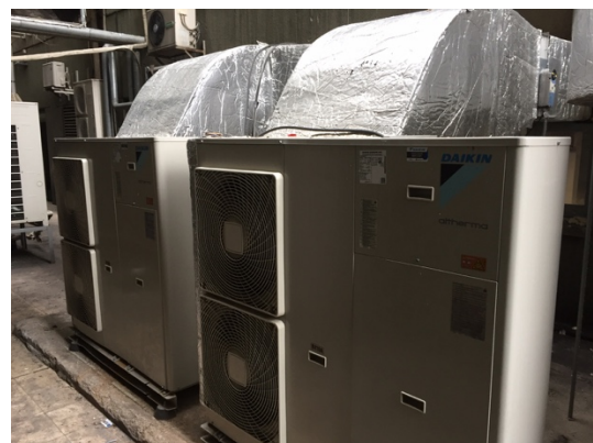
Fig. 2. Air-to-Water Heat Pumps (per unit 16 kW) of the facility.
