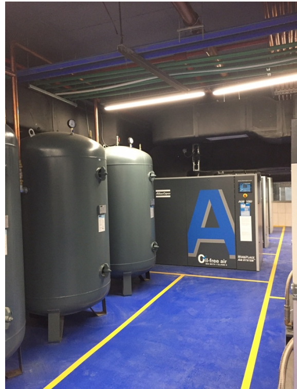
Fig. 1. Location of Oil-Free Air Compressors (center) and Air Tanks (left).
