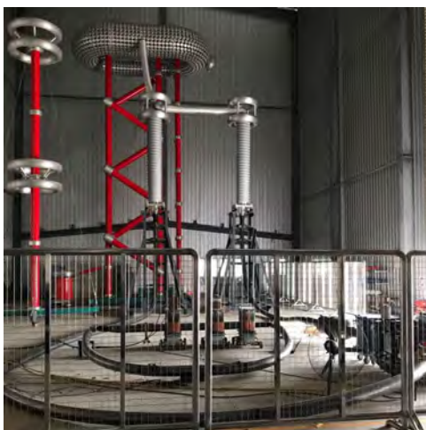
(b) Test circuit on site
