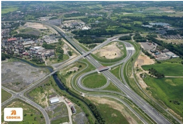
Photo. 1. A view of Piekary junction on highway A-1, constructed on complicated mining terrain (GDDKiA data [20]).
