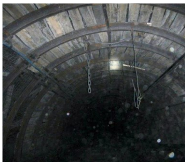
Fig. 11. Fragment of the belt entry state at an experimental site.
