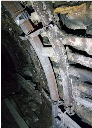
Fig. 14. An example of ŁP8/V29 steel arch support section(photo P.Ficek).
