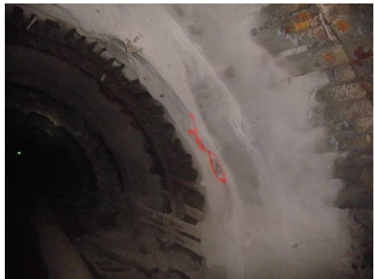
Fig. 15. An ŁP8/V29 steel arch support section covered with shotcrete layer (photo P.Ficek).
