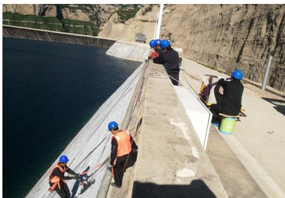
Figure 2. Field inspection of concrete anti-seepage panels
