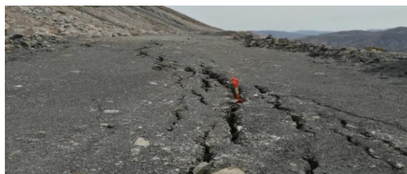
Figure. 2 Tensile cracks at the front edge of the dumping site top
