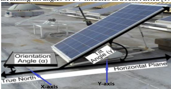
Fig. 1. The tilt and orientation angles of a PV module [20]
