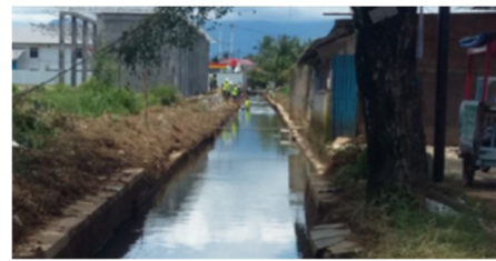
Fig.10. The refinement of the drainage canal
