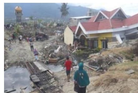
Fig.2. Sinking house in Bolora Housing due to earthquake resulting liquefaction 2018 [6].
