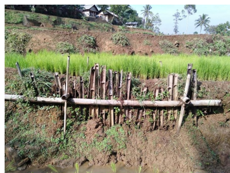
Fig. 9. " Talutug " = Local Wisdom in Structural Mitigation of Landslides
