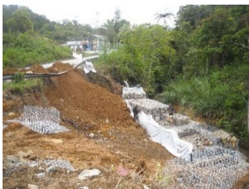
Fig.7a. The gabion retaining wall during construction
