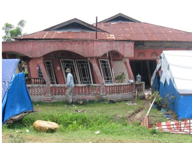
Fig. 1. Damage to houses and government buildings due to the ground amplification during the 30 September 2009 earthquake [4].
