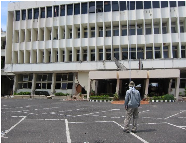
Fig. 2. Damage to government buildings and an embankment road due to liquefaction induced by the 30 September 2009 earthquake [4].
