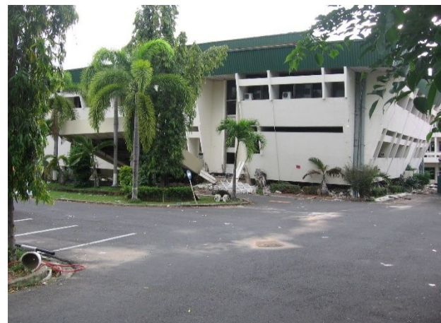
Fig. 1. Damage to houses and government buildings due to the ground amplification during the 30 September 2009 earthquake [4].
