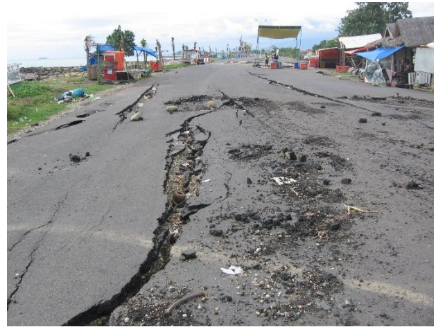
Fig. 2. Damage to government buildings and an embankment road due to liquefaction induced by the 30 September 2009 earthquake [4].
