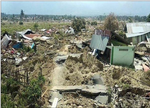
Fig 4. Conditions after liquefaction in Petobo
