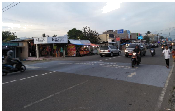
Fig. 4. Tsunami safe zone road markings on Alai – By-pass roads
