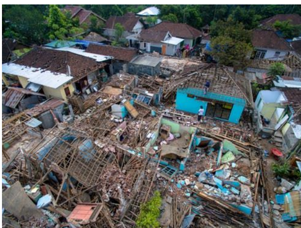
Fig. 1. The Damage in Lombok earthquake 2018 [2].
