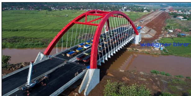
Fig. 9. Kalikuto Bridge during Loading Test (Picture by: PT. Waagner Biro Indonesia)
