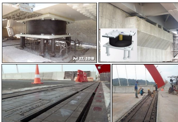
Fig. 8. Documentations of LRB and SFX Joint on site
