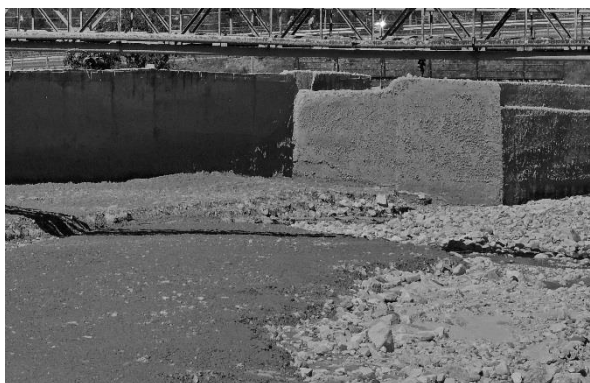
Fig. 5. Section of the mudflow tray with mud deposits 2017 (photo by M.D. Dokukin 22.08.2017)
