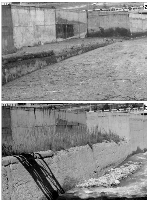
Fig. 4. Left wall of the mudflow tray in the middle of section №2: a – 04.08.2011, b – 31.07.2014 (photographs by M.D. Dokukin, view from pedestrian bridge)
