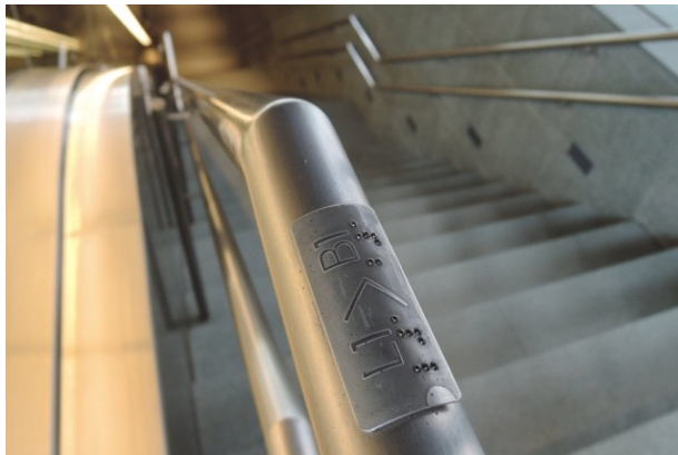
Fig. 5. Brail to indicate the way in the subway
