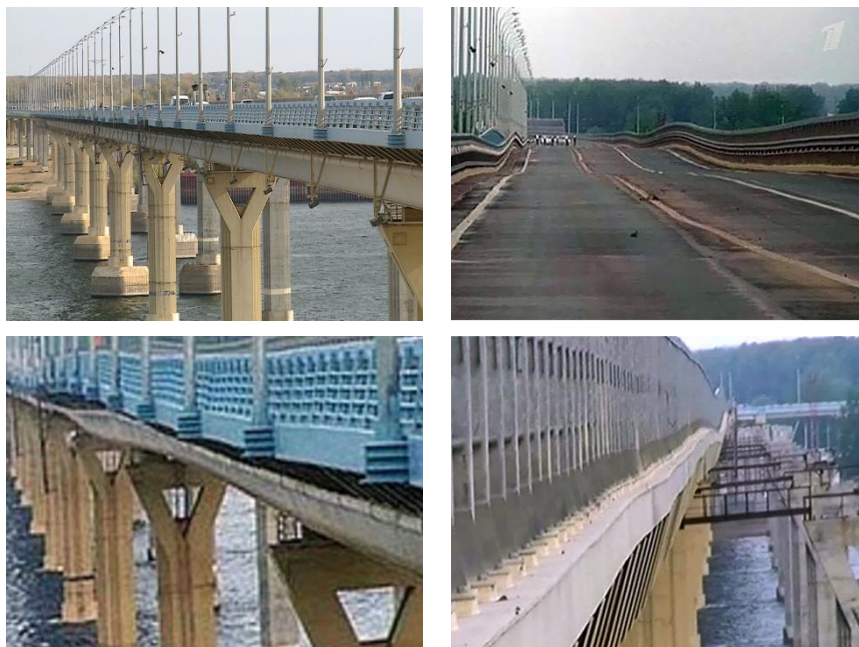
Fig. 2. Volgogradsky Bridge oscillations (the bridge before and during a period of intense oscillations).
