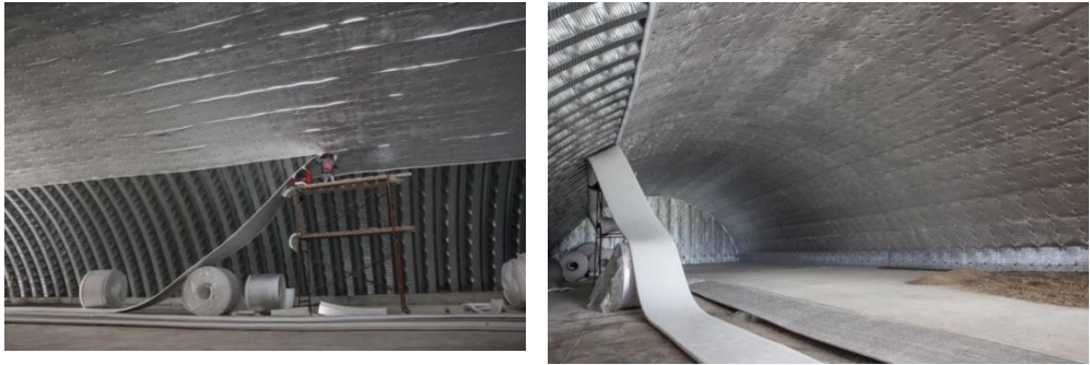
Fig. 3. Installation of the insulating coating of a hangar.
