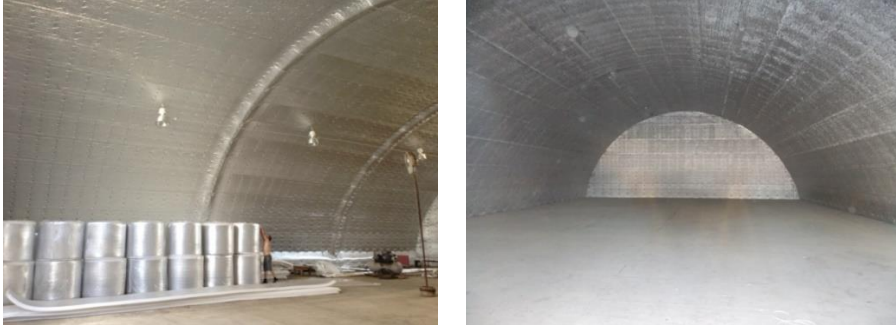
Fig. 5. Insulation of a frameless structure. Covered stockyard.
