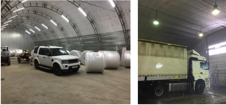
Fig. 7. Interior of heat-insulated parking areas.
