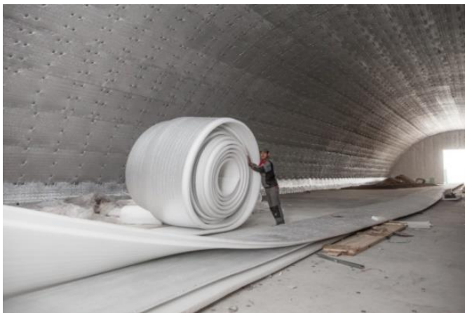
Fig. 2. Preparation of a roll of metallized polyethylene foam.
