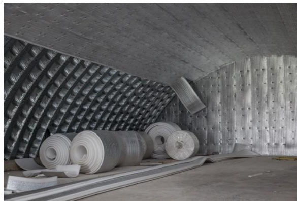
Fig. 6. Insulation of the end face of a vegetable storehouse.
