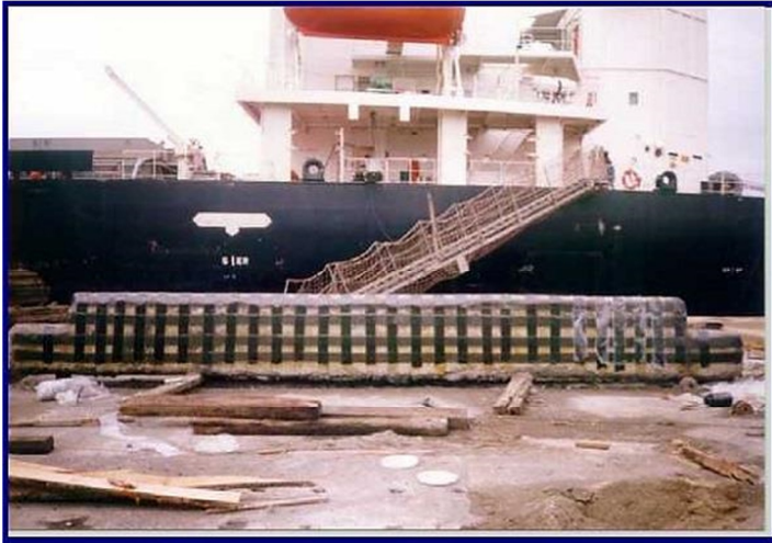
Fig. 4. The edge beam during the carbon stripes adhering process.
