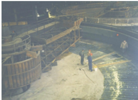
Fig. 7. Overall view of the coagulation unit during the strengthening.
