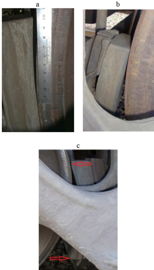
Fig. 2. Pictures of the wedge dual wear of the brake pad in operation: a – measurement of the length of harmful wear; b – interaction of the upper end with the rolling surface of the wheel during movement of the car; c – abnormal clearance between the pad and the wheel.
