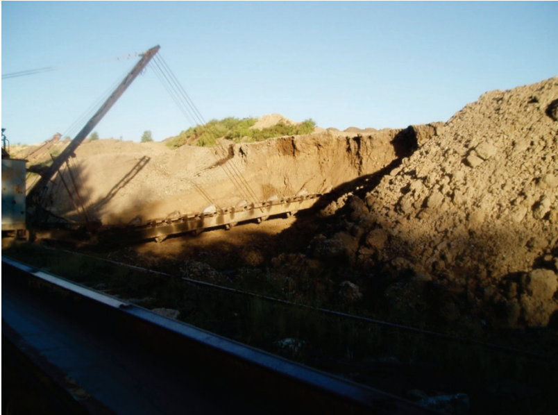
Fig. 4. Bucket excavator, Source: Ing. J. Fiala 2019.
