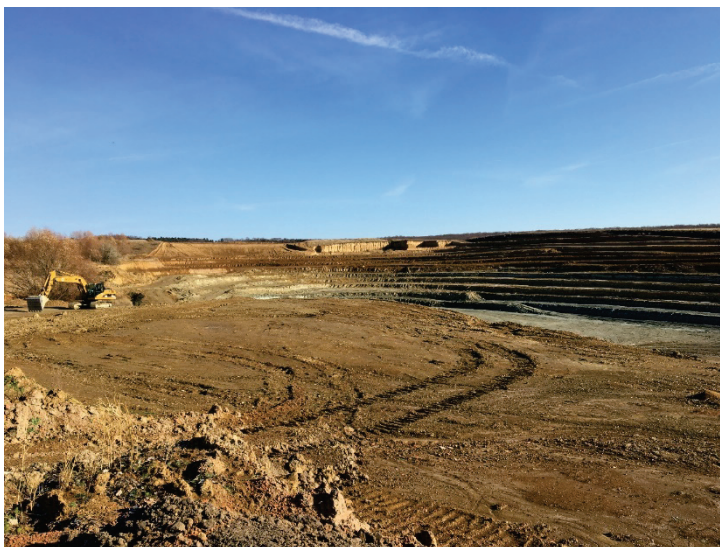
Fig. 2. Excavation premise of surface mining, Source: Wienerberger.
