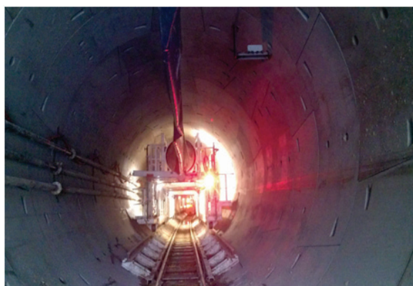
Fig. 4. Finished high-quality tunnel lining (Tashkent-2018).
