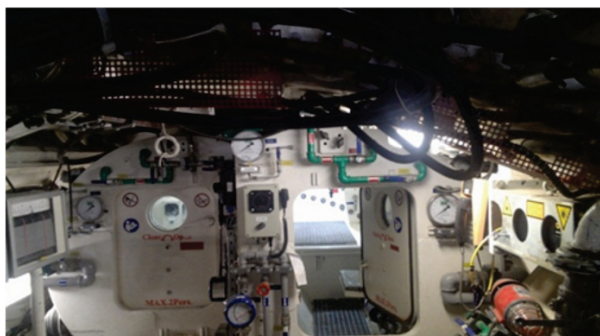
Fig. 2. Airlock shield chamber (Tashkent-2018).
