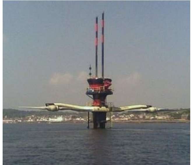
Fig.4 – MHK turbine Seagen with rotors raised. Image from upload.wikimedia.org/wikipedia/commons/e/e1/Seagen_raised.jpg
