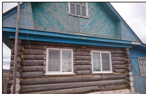
Fig. 5. The location of the MiniMate Plus seismic recorder near a one-story barrack type residential building (1 Berezovaya St., Maly Berdyash settlement) - p. 3.
