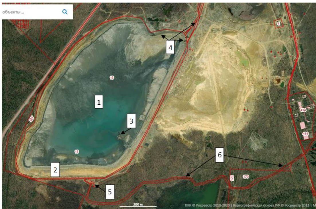
1 – basin (settlement pond), 2 – embankment, 3 – drainage sump, 4 – pulp lines, 5 - pumping station, 6 – catch drain of accidental clarified water discharge
