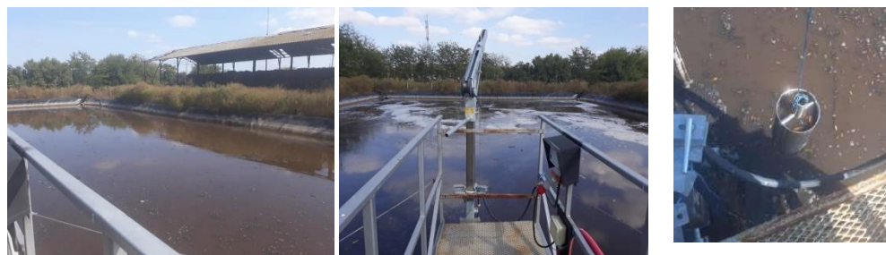
Fig. 2. Lagoon for wastewater storage, mechanical stirrer and wastewater sampling
