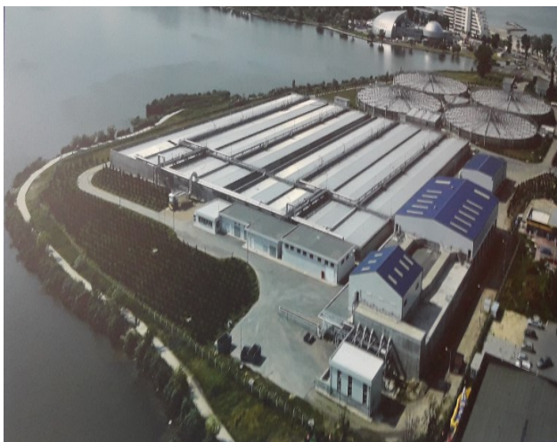
Fig. 1. The sewage treatment plant in North Constanta –View after covering the objectives that gave repellent gases
