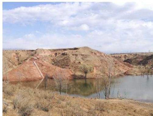
Fig. 3. Reality images of river and earth dam
