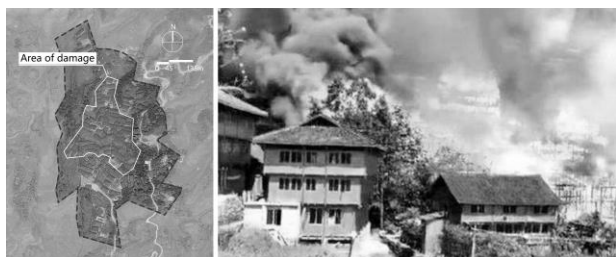
Fig. 2. Fire damage area and scene photos of Xiaozhai Village
