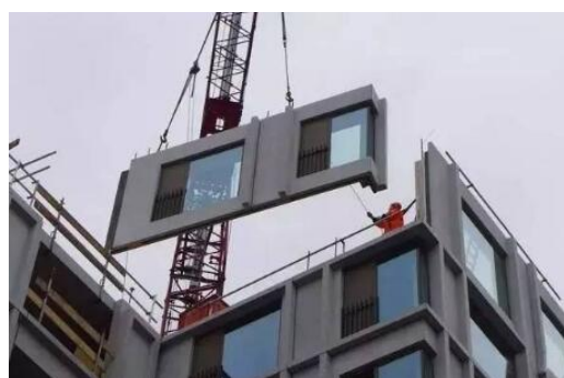
Fig.1. Construction site of prefabricated assembly components
