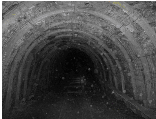
Fig. 7. An illustration of a mine working state according to the recommended fastening scheme.
