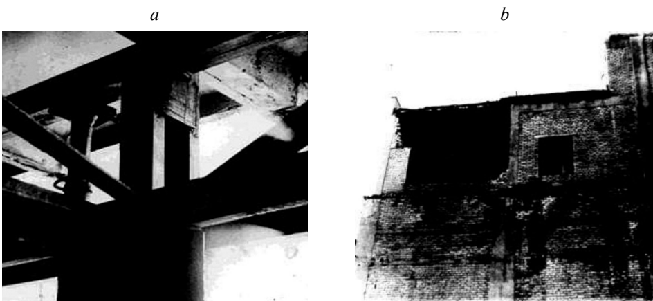
Fig. 5. The lifting supporting beam and hydraulic shaft lining (a) and completely unmounted load-bearing wall of the building of the bunker (b).
