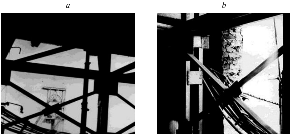
Fig. 4. The main supporting beam, raising by shaft lining upwards (a) and the rack of the supporting panel and unmounted wall (b).
