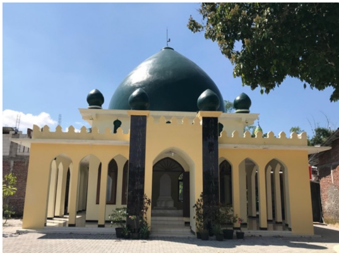
Fig. 2. The Dome Tomb of Sayid Luhung Alwi after renovated (Source: Photo by Rabith Jihan Amaruli, 2020).
