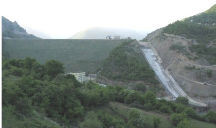
Fig. 5. View of Zhinvali Earth Dam from the tailrace
