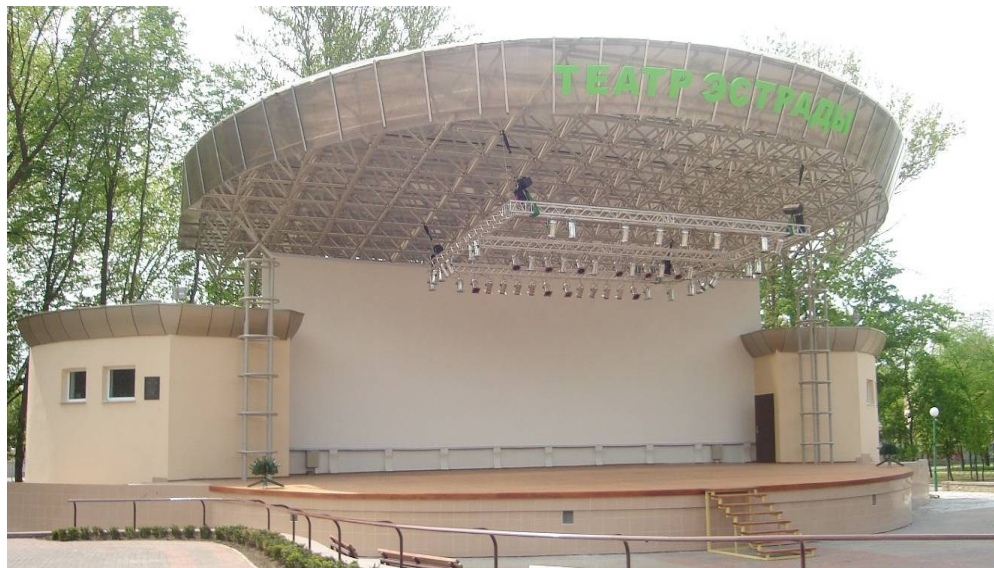
Fig. 1. General view of the structural slab in Brest.
