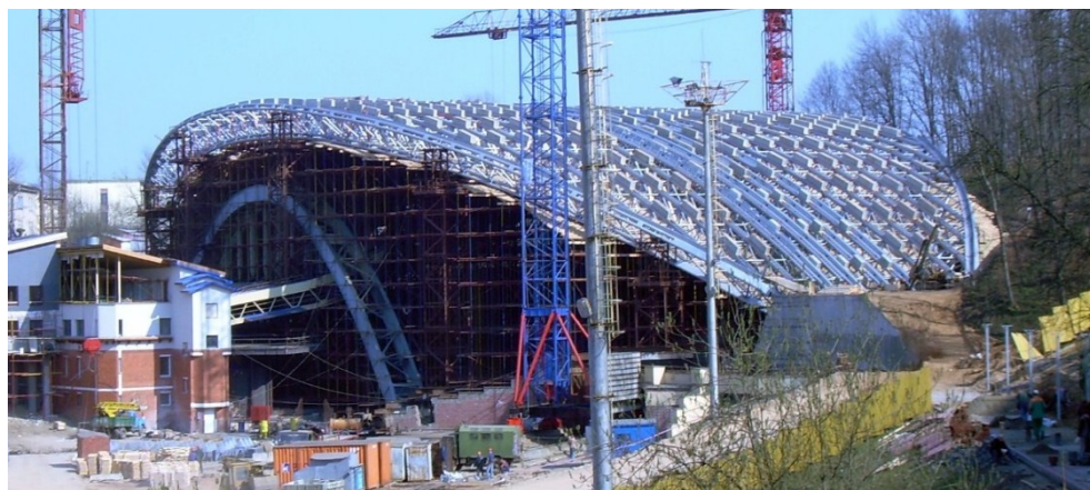
Fig.5. General view of the roof under test load.
