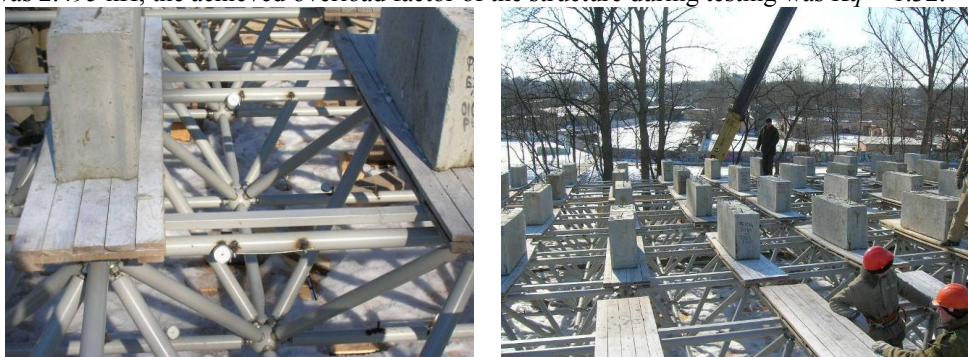
Fig.2. Testing the structural plate by static load.
