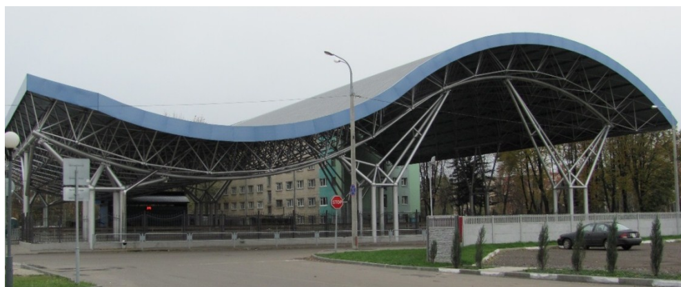
Fig. 7. General view of the ice rink roof in Gomel.
