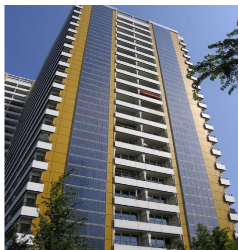
Fig.1. Photovoltaic systems: b) Energy supply of high-rise buildings with a connection to the city network.
