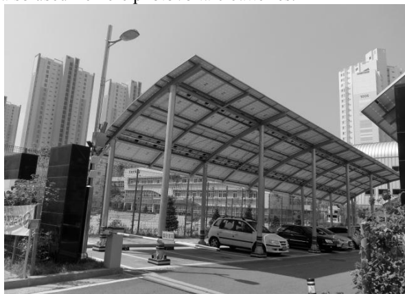
Fig.1. Photovoltaic systems: a) PVB as a car sun protection coating parking in the form of a fragment of a cylindrical surface.
