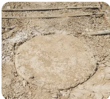
Fig.6 comparison between self-made slurry and new slurry material in drilling to pile surface
